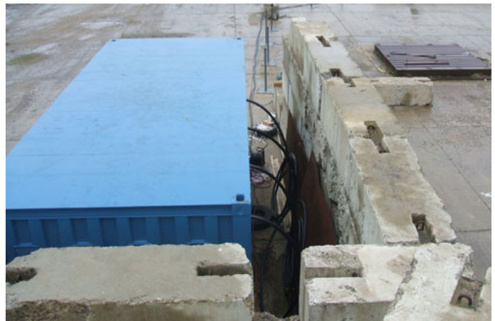
Fig. 25 The container is protected with concrete blocks
